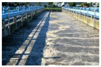
Insufficient oxygen supply results in incomplete decomposition of harmful substances and thus insufficient cleaning performance. In the worst case, statutory limit values might be exceeded.
