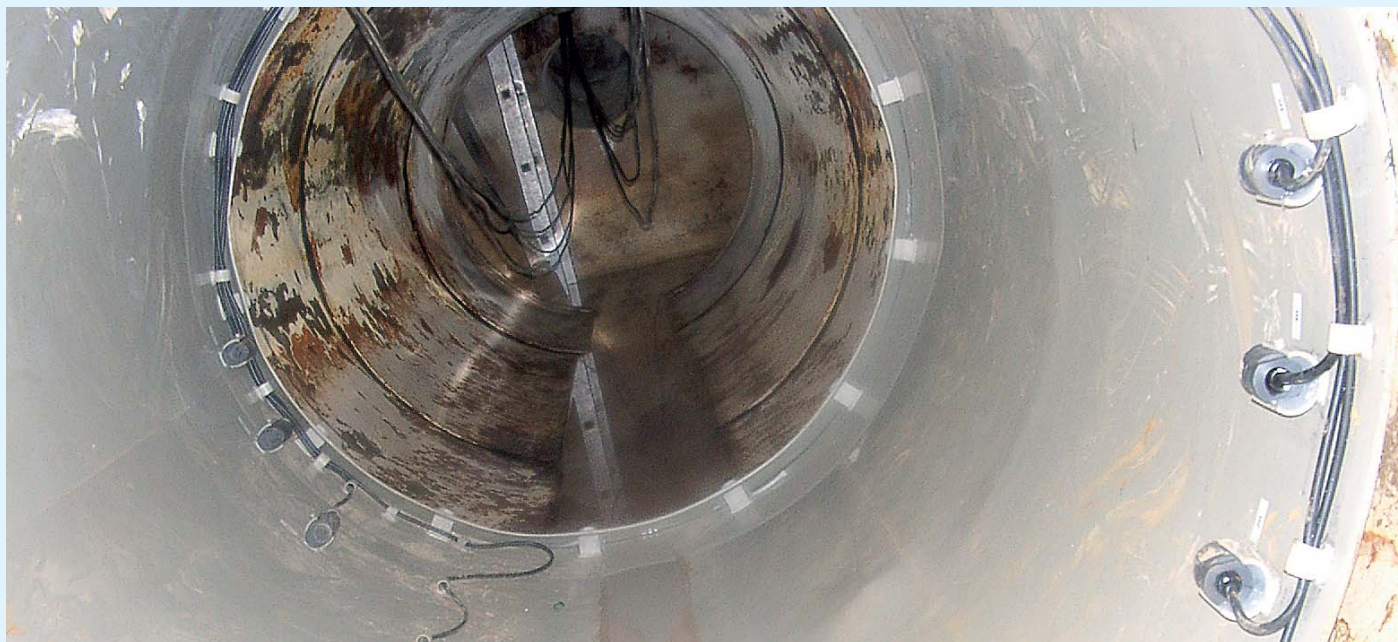
THE ASSEMBLY RING: on entry into the narrow wastewater inspection manhole.
